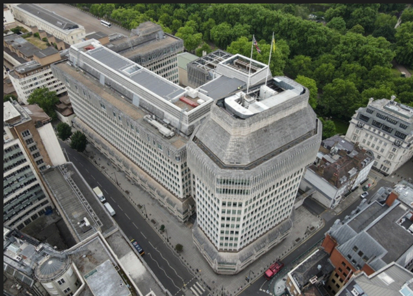
ROOF & FACADE INSPECTION, MINISTRY OF JUSTICE, PETTY FRANCE, LONDON
