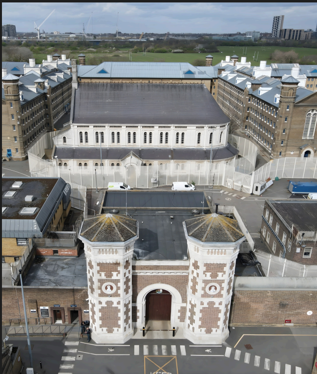
CONDITION SURVEY, HMP WORMWOOD SCRUBS, LONDON
