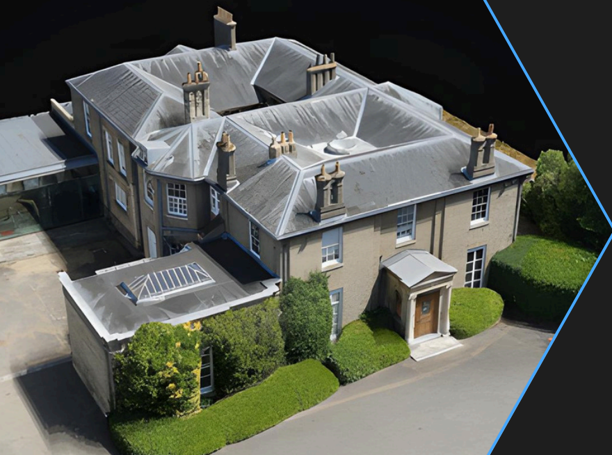
HISTORIC ENGLAND HEADQUARTERS, CAMBRIDGE
