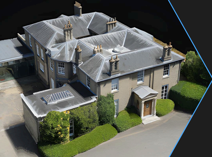
HISTORIC ENGLAND HEADQUARTERS, CAMBRIDGE
