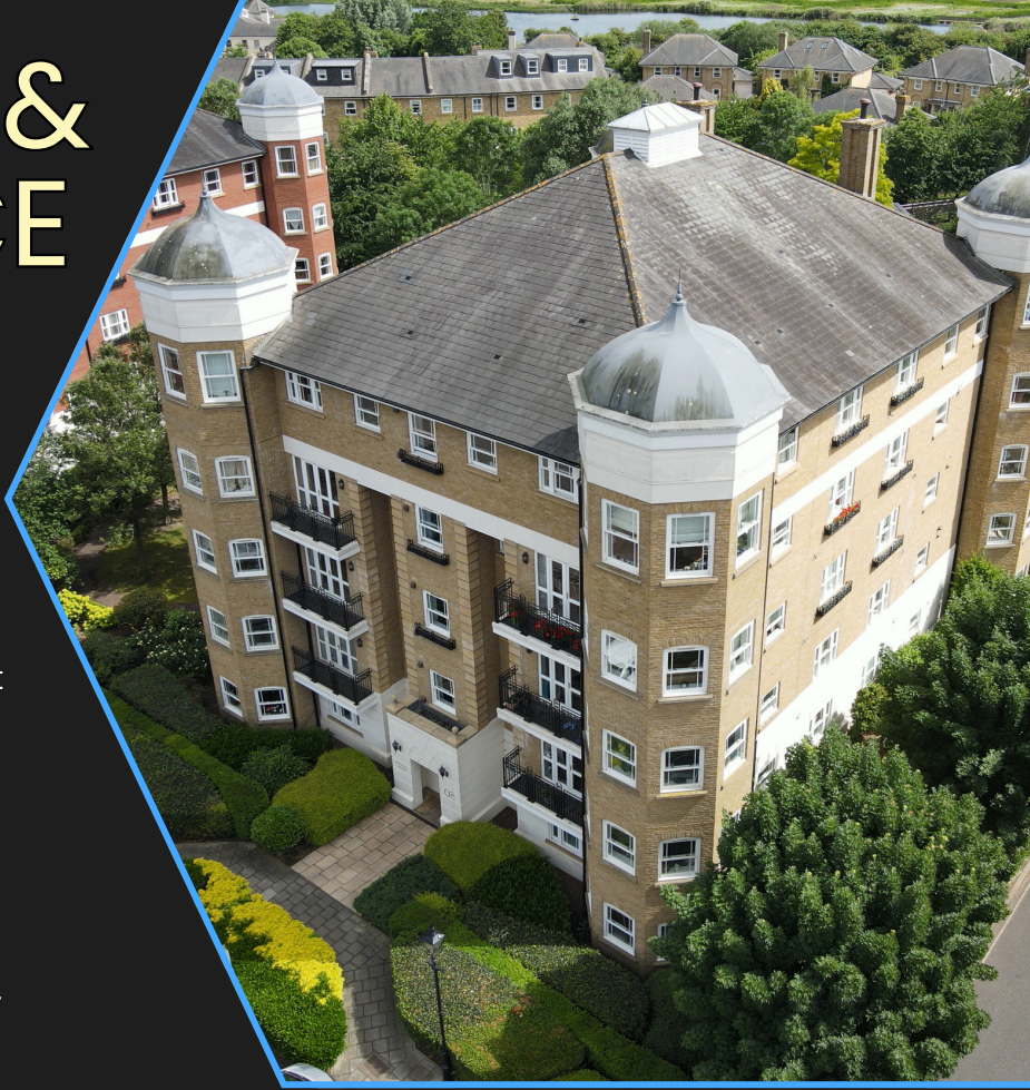
3D CONDITION SURVEY, CLAYTON HOUSE HARRODS ESTATE, LONDON
